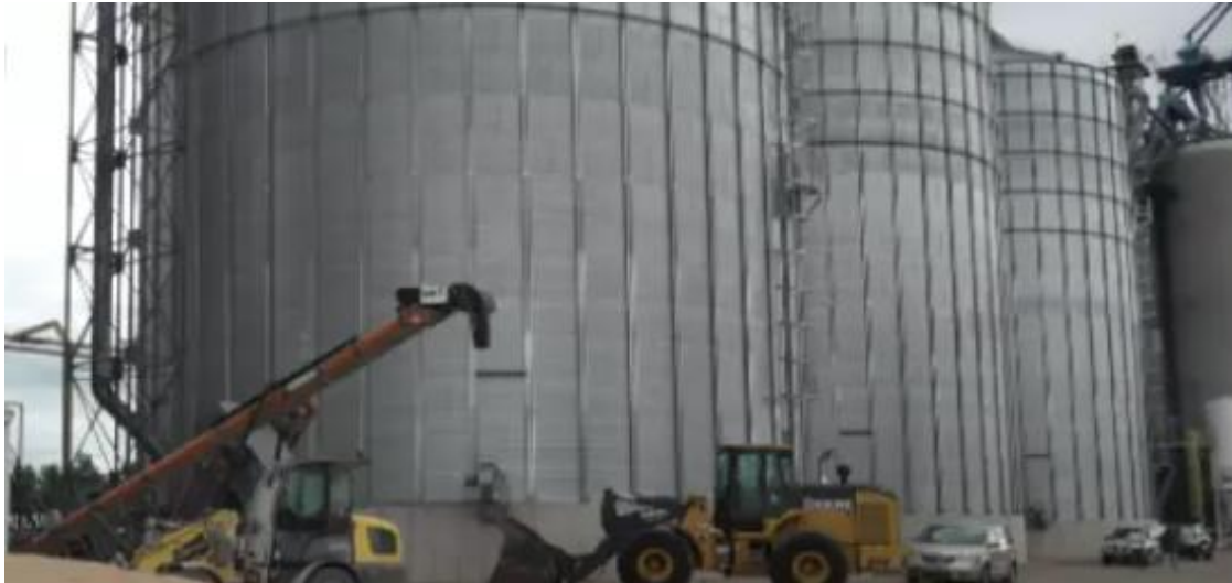
Figure 11. Cleaning area of bin
